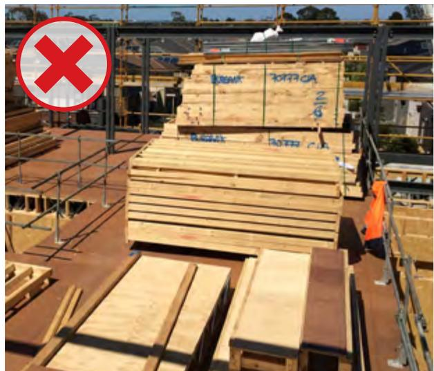
Cassette floors should not be loaded with pre-nailed wall frames more than 1.5m deep
